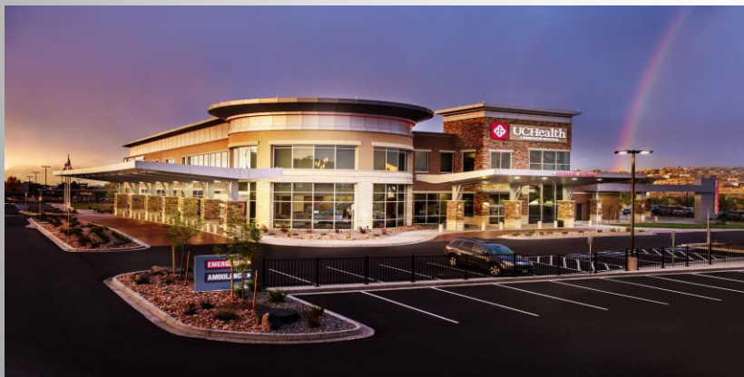
Grandview Hospital- Colorado Springs
